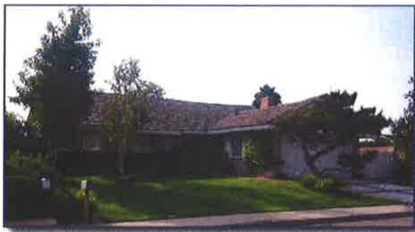
Example of California Ranch Architecture
